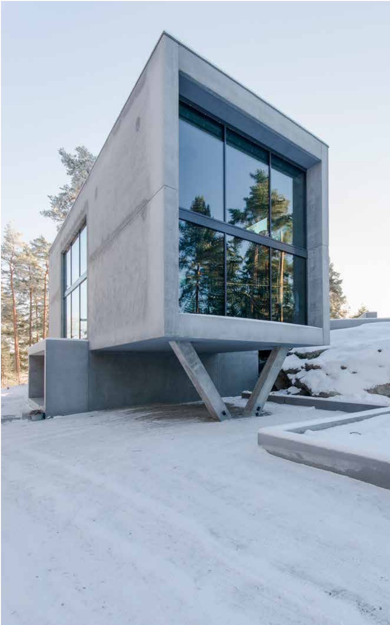
The large areas of glass on the gable ends and long sides of the house couple the interior spaces with the natural surroundings.
